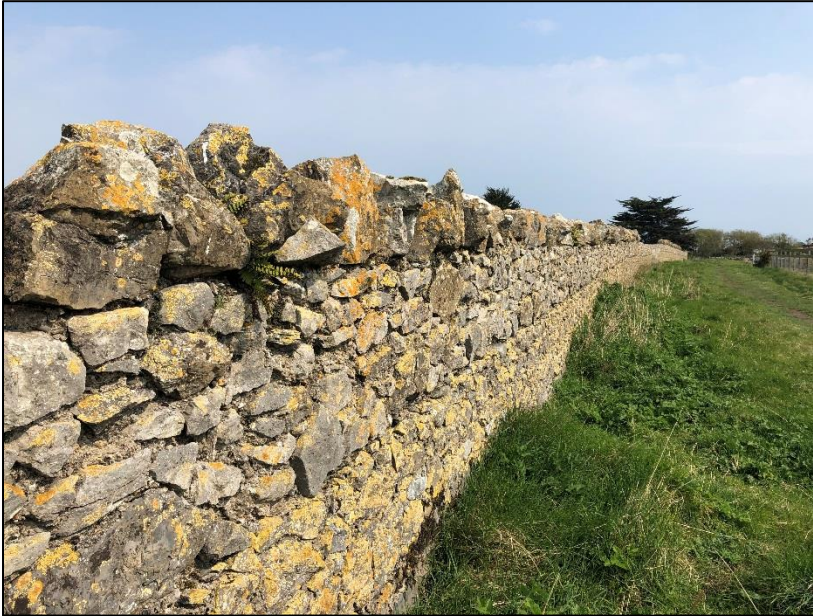
Plate4: Stonewall present on site (April 2019).
