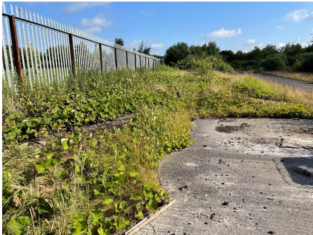
Plate 2: Winter heliotrope looking north along the western boundary
