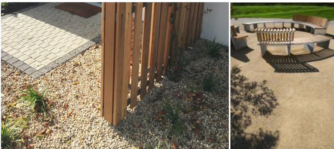
Figure 11: Range of hard landscape finish details (from left to right): permeable gravel detail, self-binding gravel.
