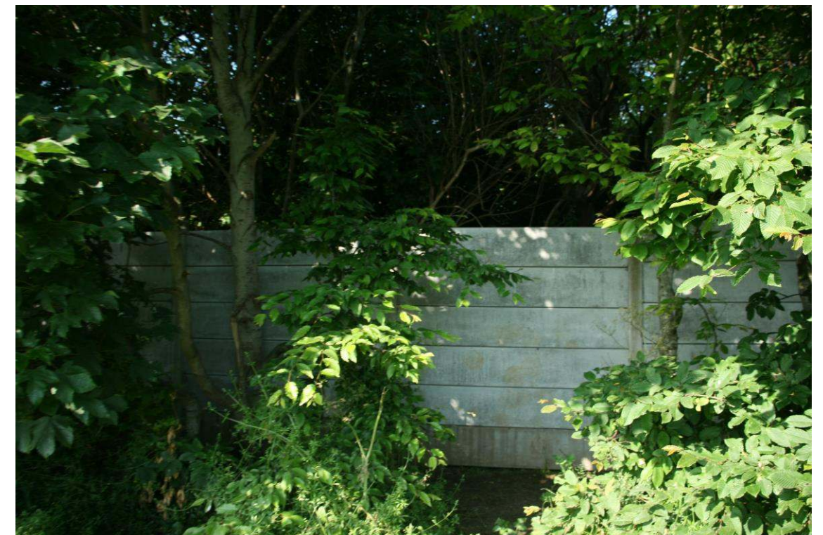
Figure 3: Photograph of the concrete post and panel fence along the southern boundary of the site.
