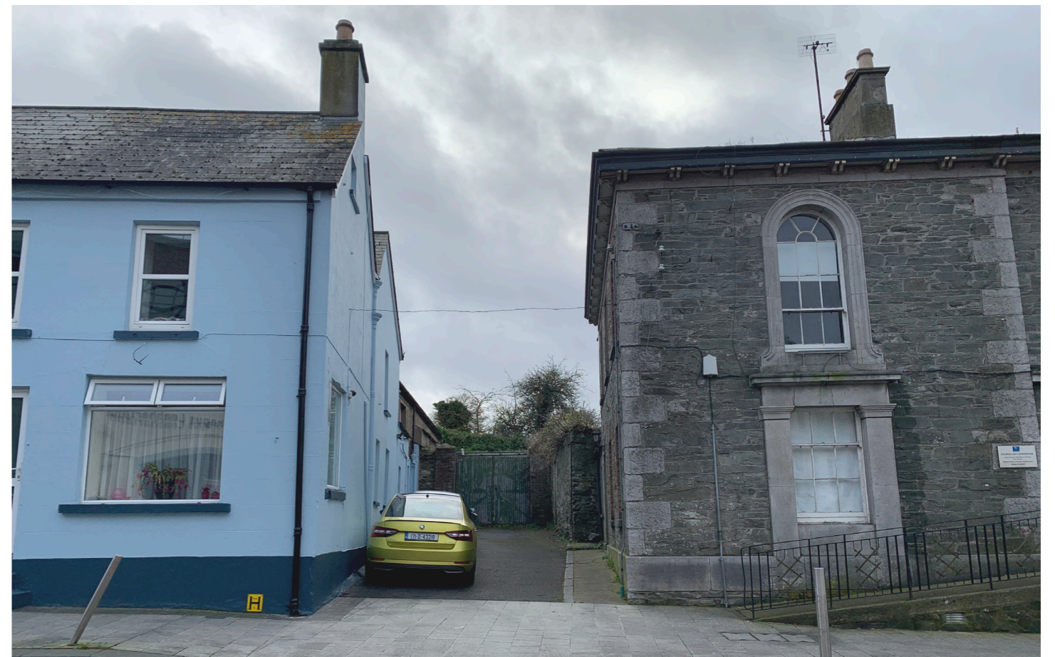
Above right: Rear of no2 Dublin Street Below right: Laneway
