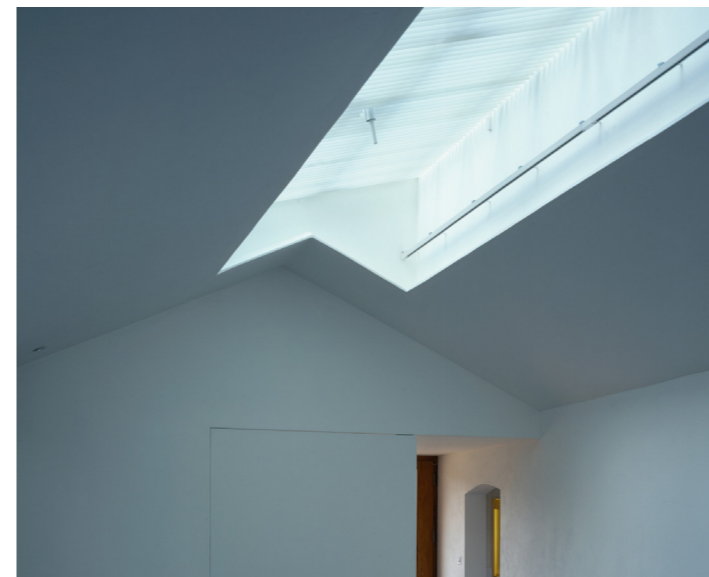
Gallery / Workshop Roof lights
