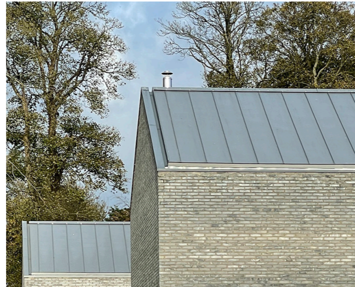
Standing seam zinc roof
