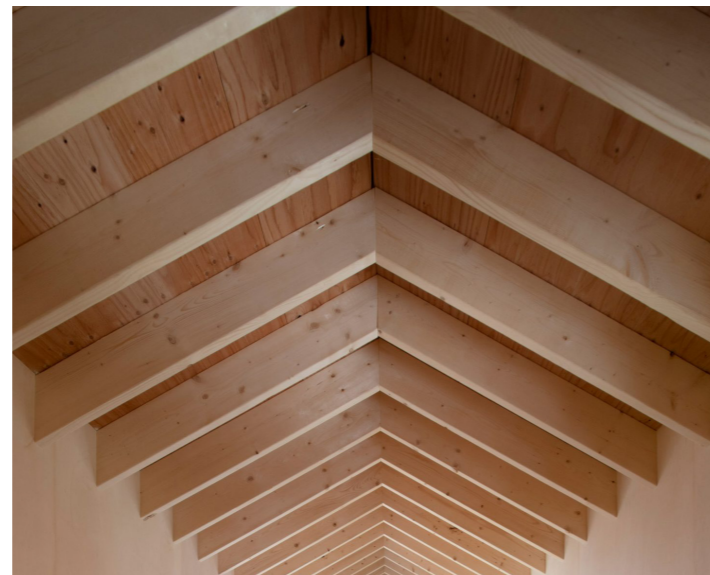
Exposed roof structure
