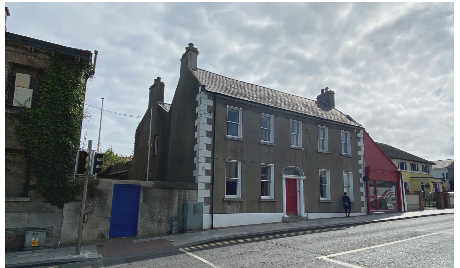
Dublin Street facade
