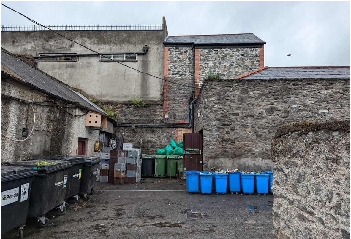
The stone structures west of the Old Couch House at Ross Cottages
