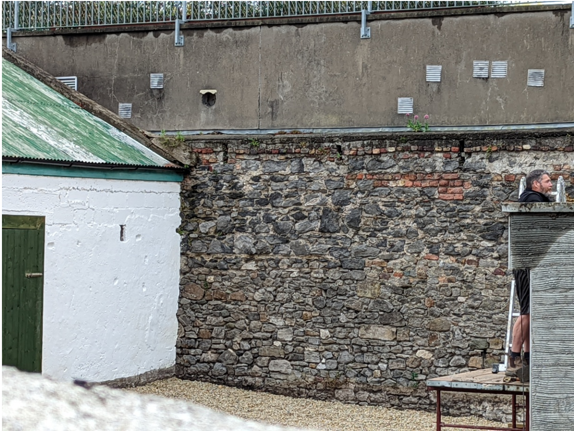
A wall in a property adjacent to the 19th century outbuilding
