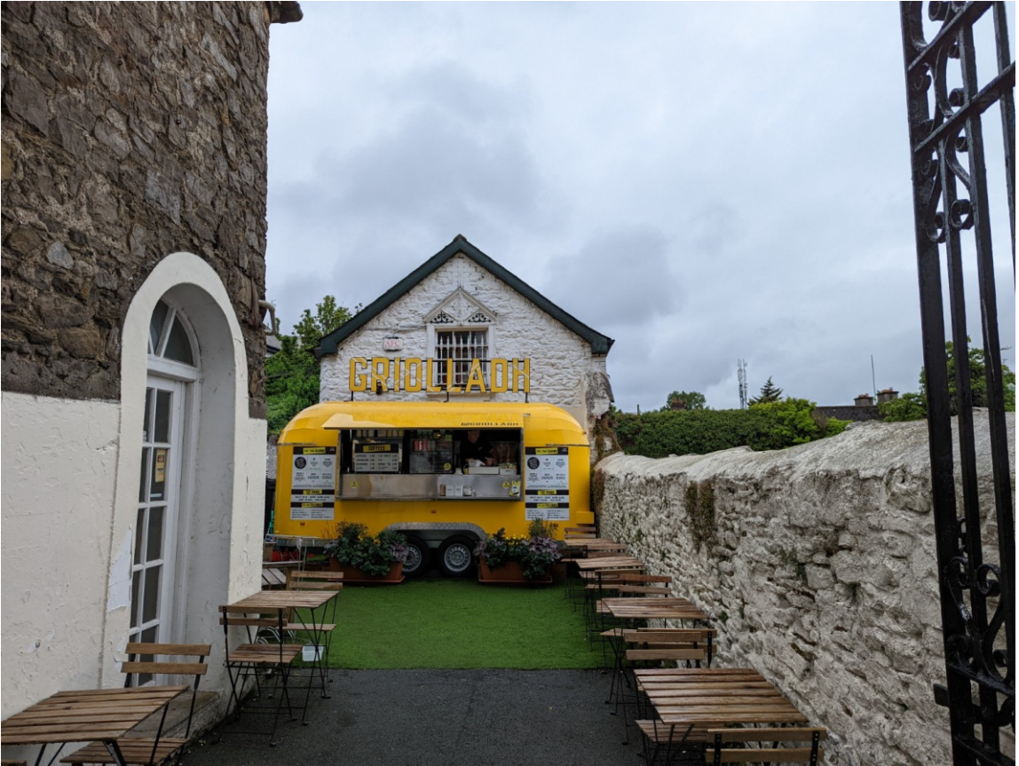
The 19th century outbuilding behind 13 New Street
