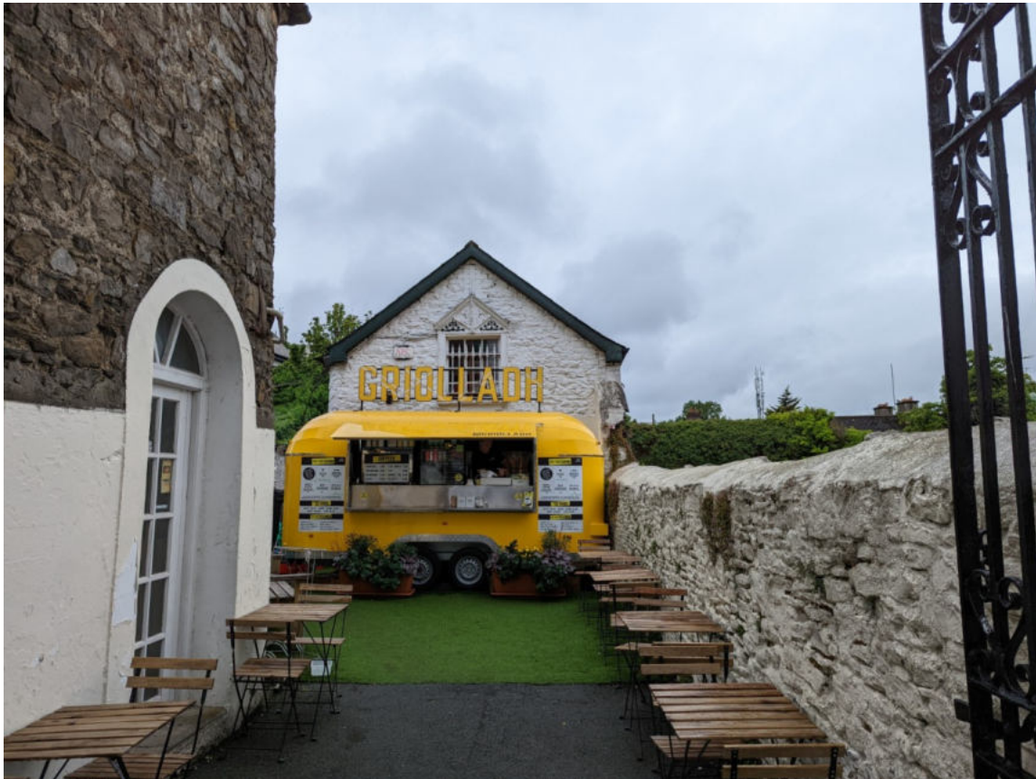
The 19th century outbuilding behind 13 New Street
