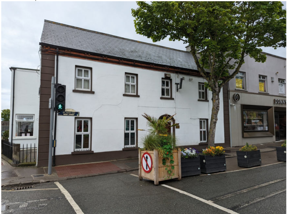
A 19th century home at the northeast corner of New Street
