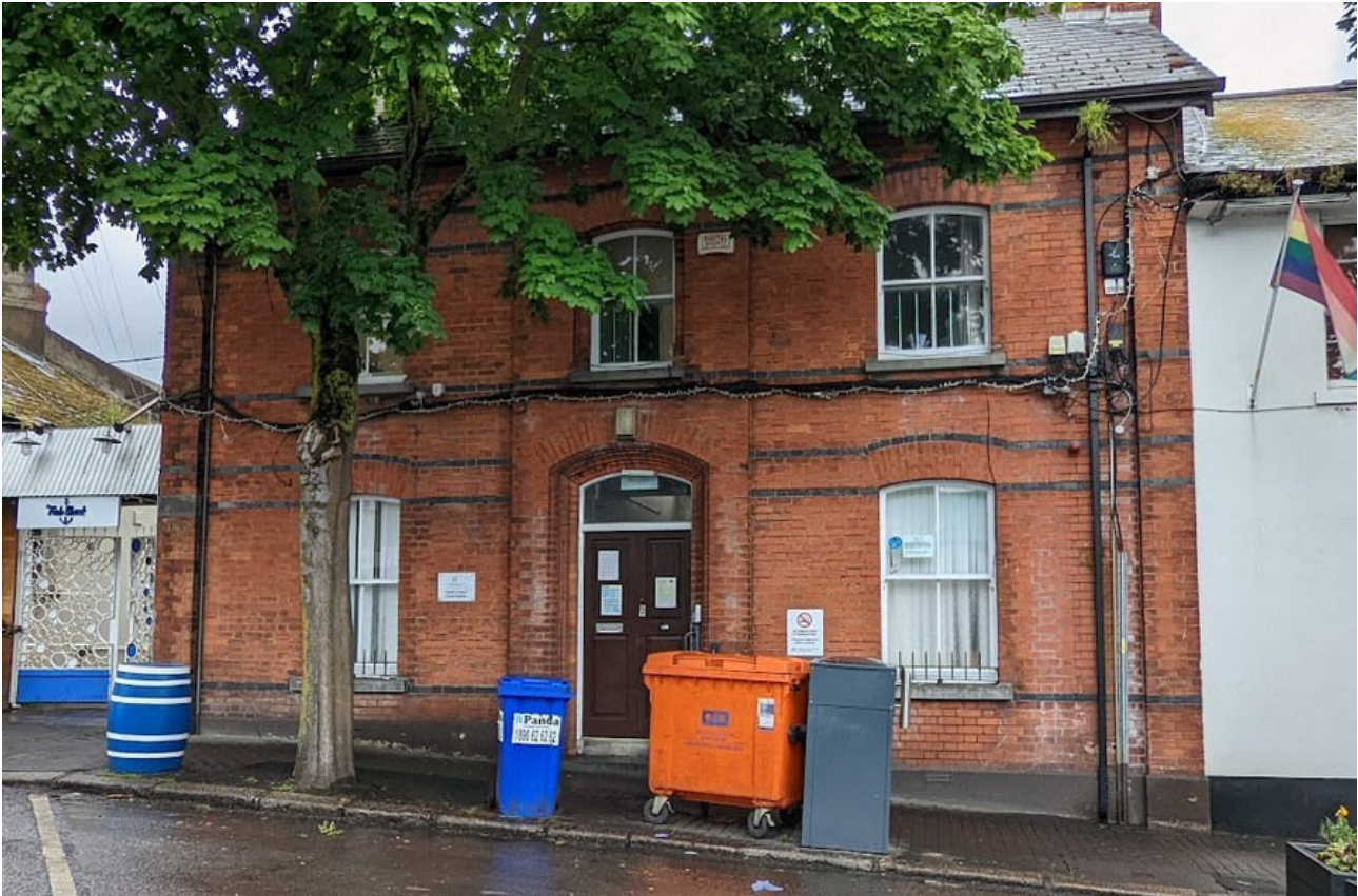
The dispensary on New Street
