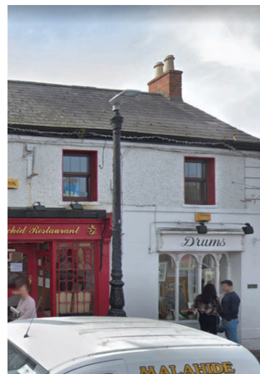
Fig. 72: New Street - 2019 - Note Lamp Standard in Place with LED fixture.
