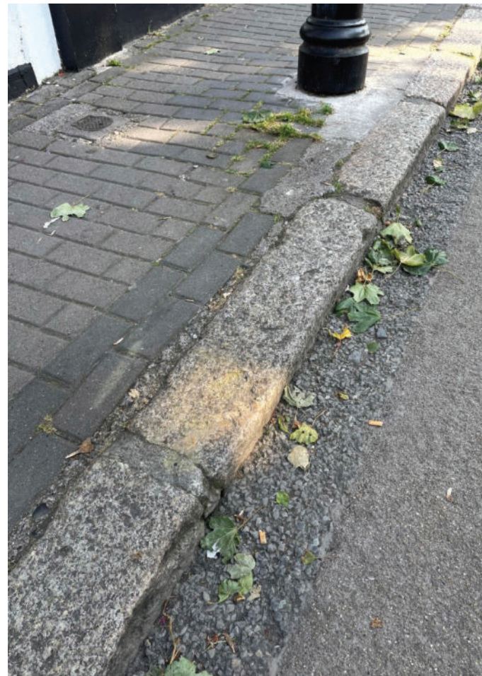
Fig. 79: New Street Existing Kerbing
