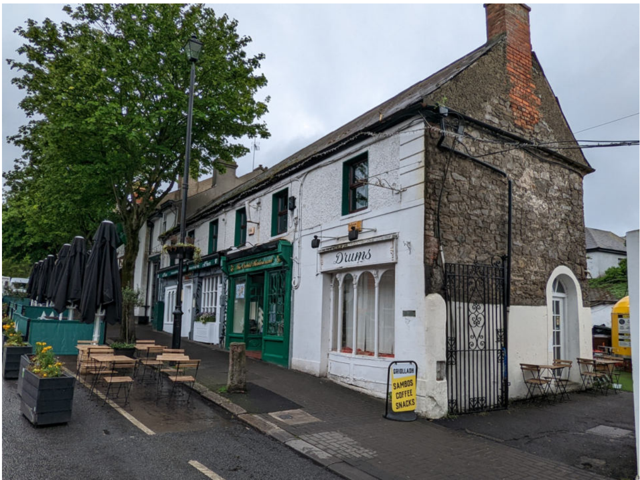
A 19th century structure with historic storefront and bowed window
