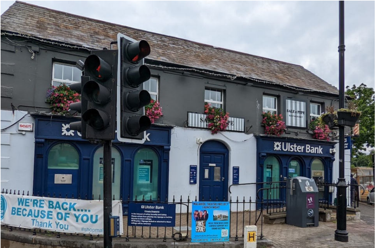
The northeastern house, now in use as a bank
