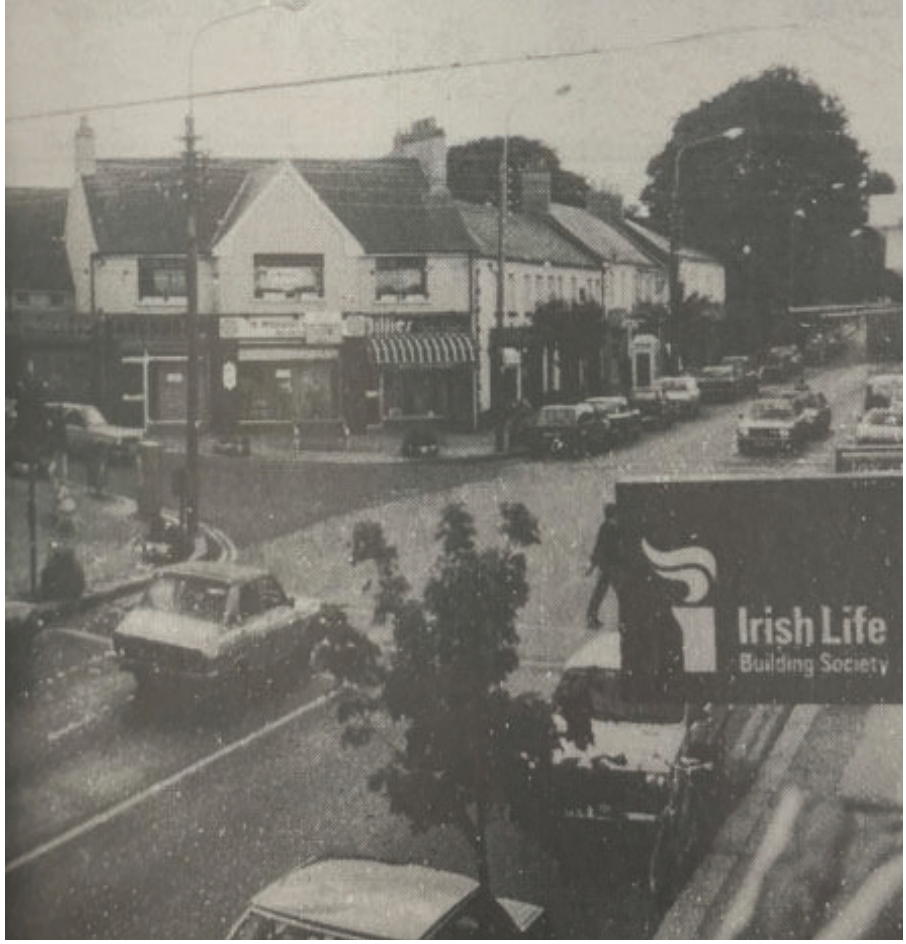
Fig. 41: The Diamond former RIC Barracks on south-east side - Image 1980s
