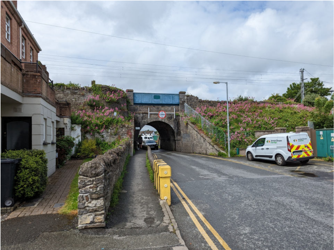
Railway station bridge on Strand Street
