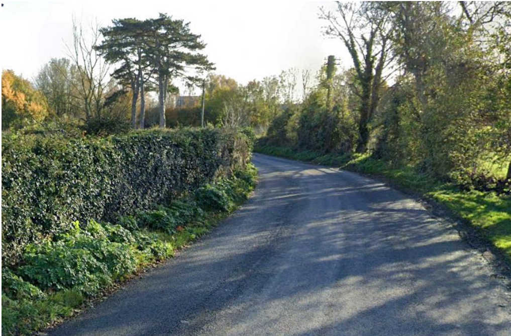
Figure 4.6 – Limited forward visibility on approach to Newtown Bridge, Balheary Road
