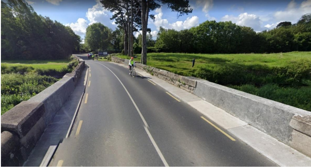
Figure 4.3 – Newtown Bridge, Balheary Road Protected Structure
