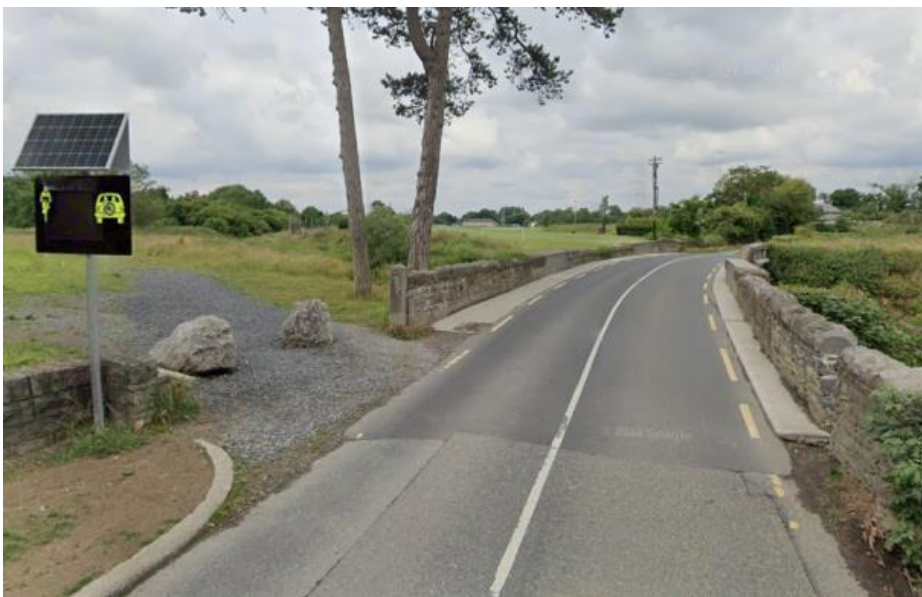
Figure 4.5 – Existing linear park pedestrian crossing with poor accessibility and poor visibility.
