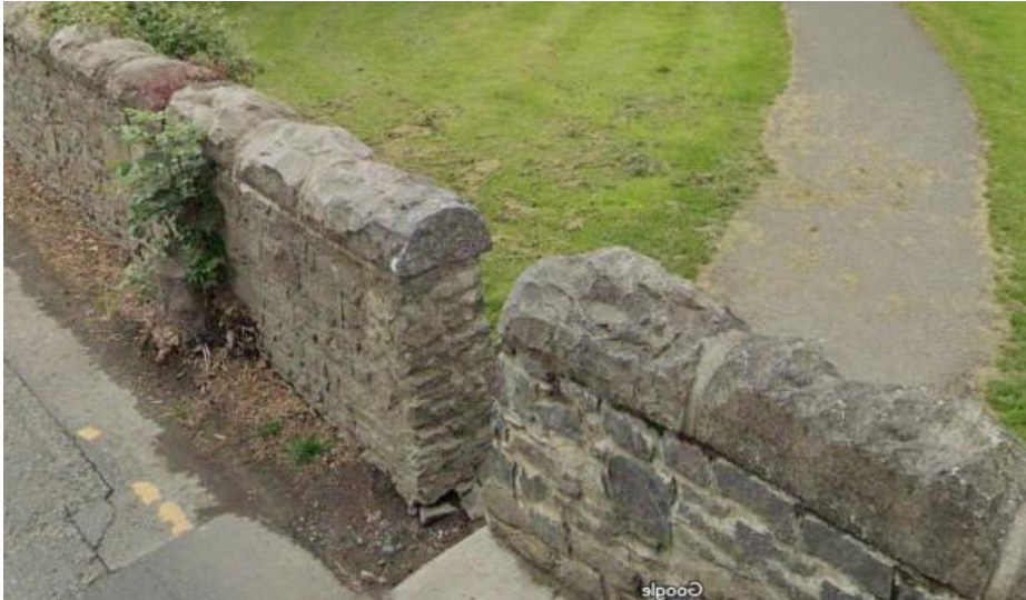
Figure 4.4 – Existing entrance to east side of linear park
