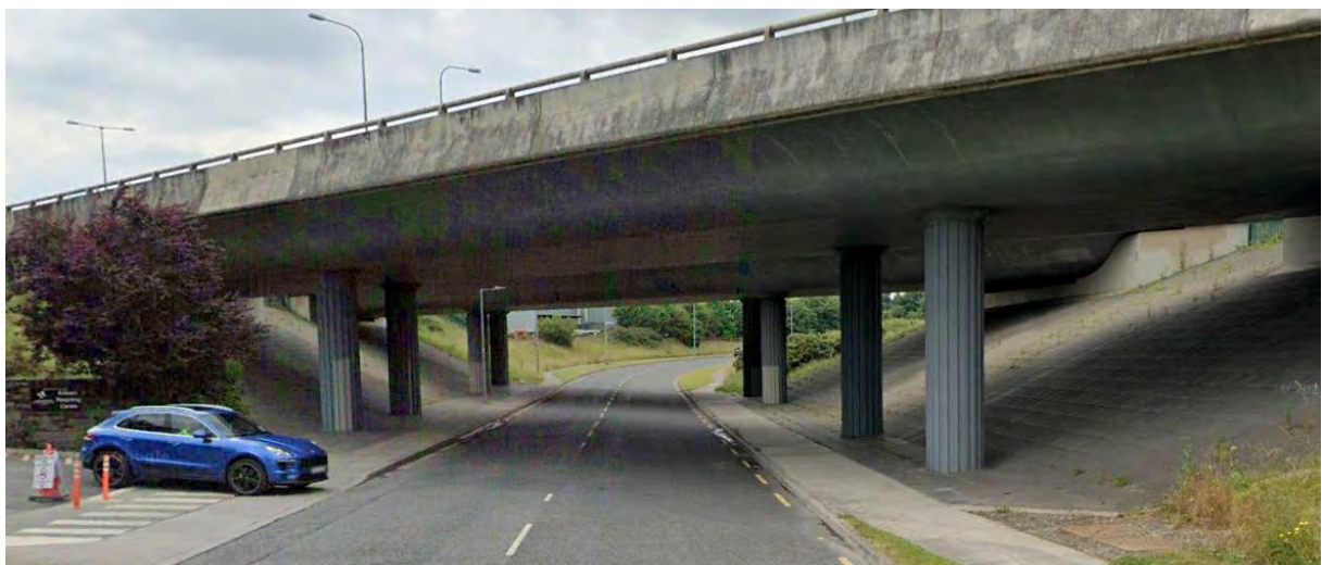
Figure 4.2 - Existing M1 Underpass
