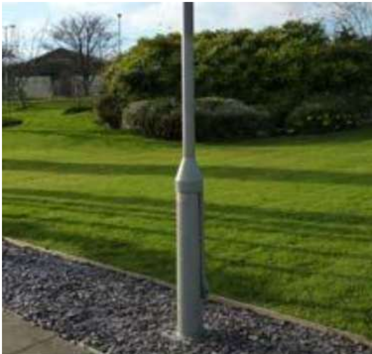
Image 5.1: Typical Base Hinged 6 meter public lighting pole:
