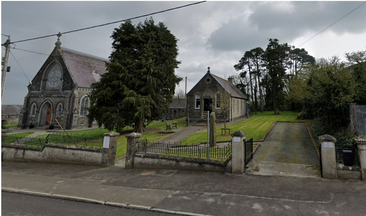
Figure 1.2 Street view of subject site (Source: Google Maps)
