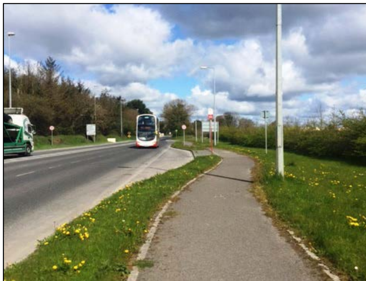
Figure 3.2 View of the Western Boundary of the Subject Lands (right) from the R135 which includes a Shared Footpath and Cycleway and Bus Eireann Bus Stop along the R135
