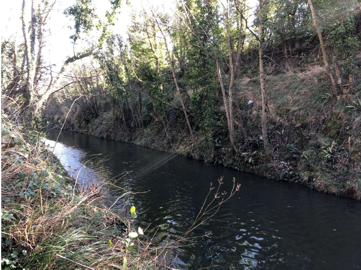
Figure 3-14: Presence of heavily vegetated overburden along the southern embankment
