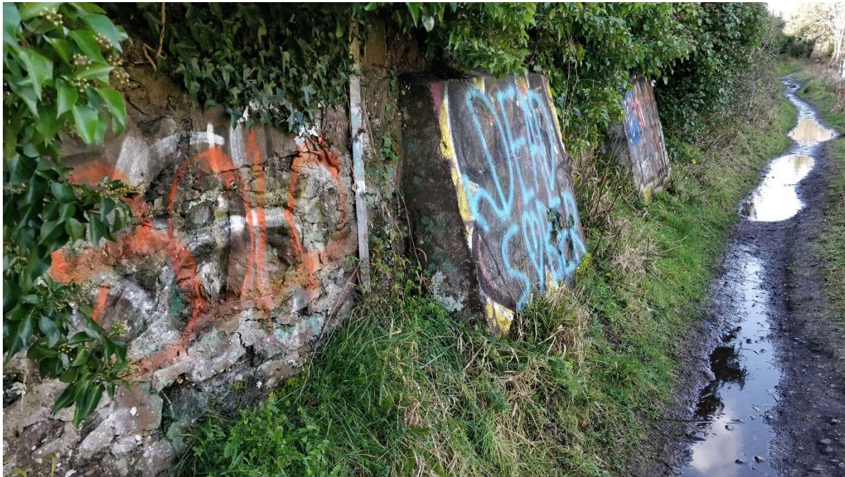
Figure 3-20: Retrofitted buttresses to support stone masonry retaining wall support railway line
