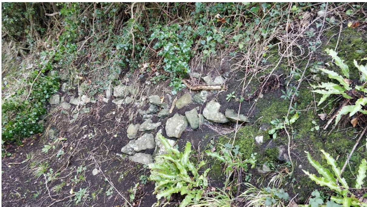
Figure 3-19: Apparent masonry retaining wall supporting Dublin-Sligo railway line
