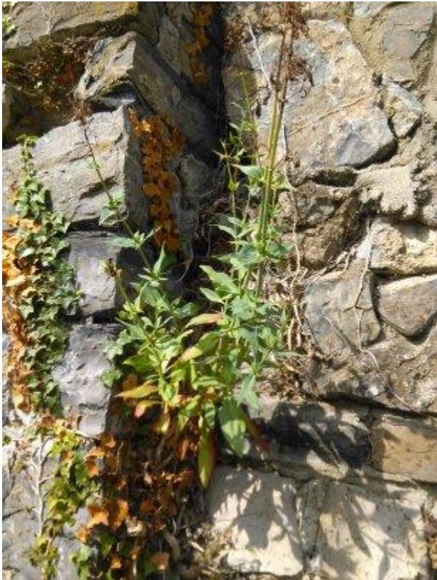
Plate 4 Red valerian ( Centranthus ruber ) can break apart stone work and damage structures.
