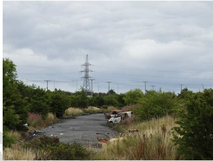
Plate 9: Eastern roadway facing north-east
