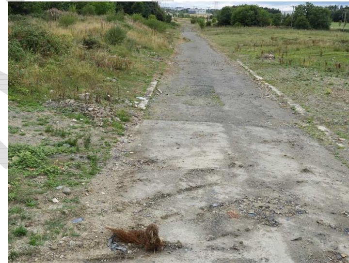
Plate 11: Western roadway, facing west
