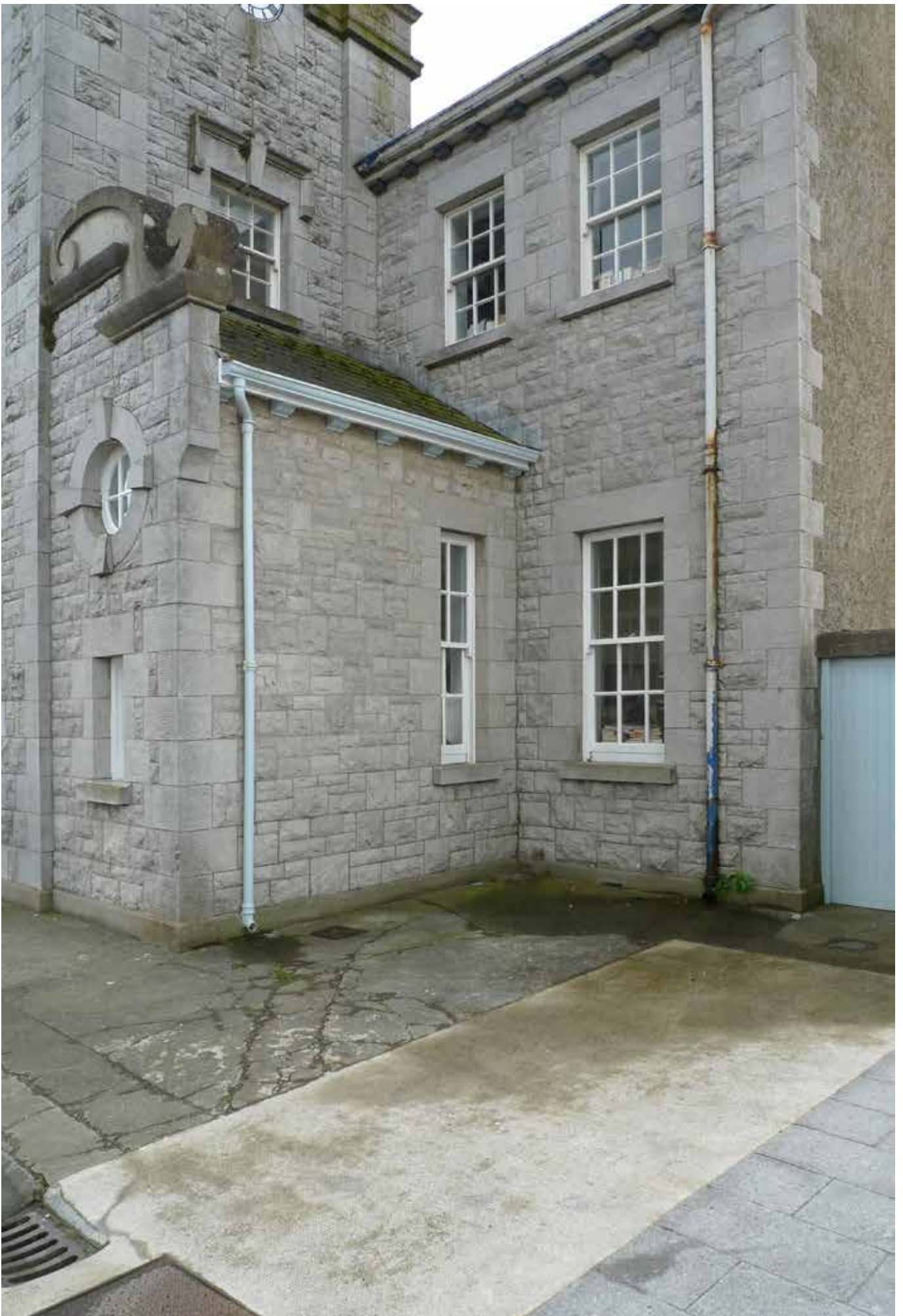
Oblique view of the northern side of the front facade of Skerries Library. Defects are evident in the rainwater goods, external painting, surface of the forecourt, surface water drainage, etc (see notes on the previous page). There is a broken vent to the ground floor sub-floor space visible below the window on the right. It is important that sub floor vents be retained, and maintained in good repair.
