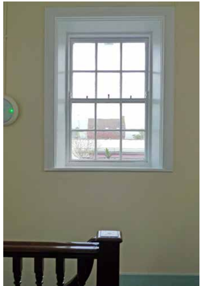
6 over 6 up and down sash window to the front of the first floor stair hall.
