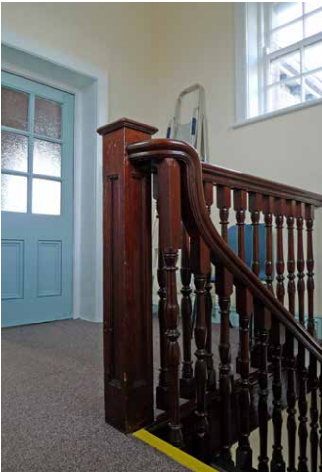
Newel, handrail and balusters at the top of the main stair.
