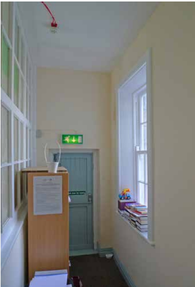
Corridor to the front of the north side of the ground floor, the exit route impeded by boxes and a bookcase. The value of an exit in this location is doubtful.
