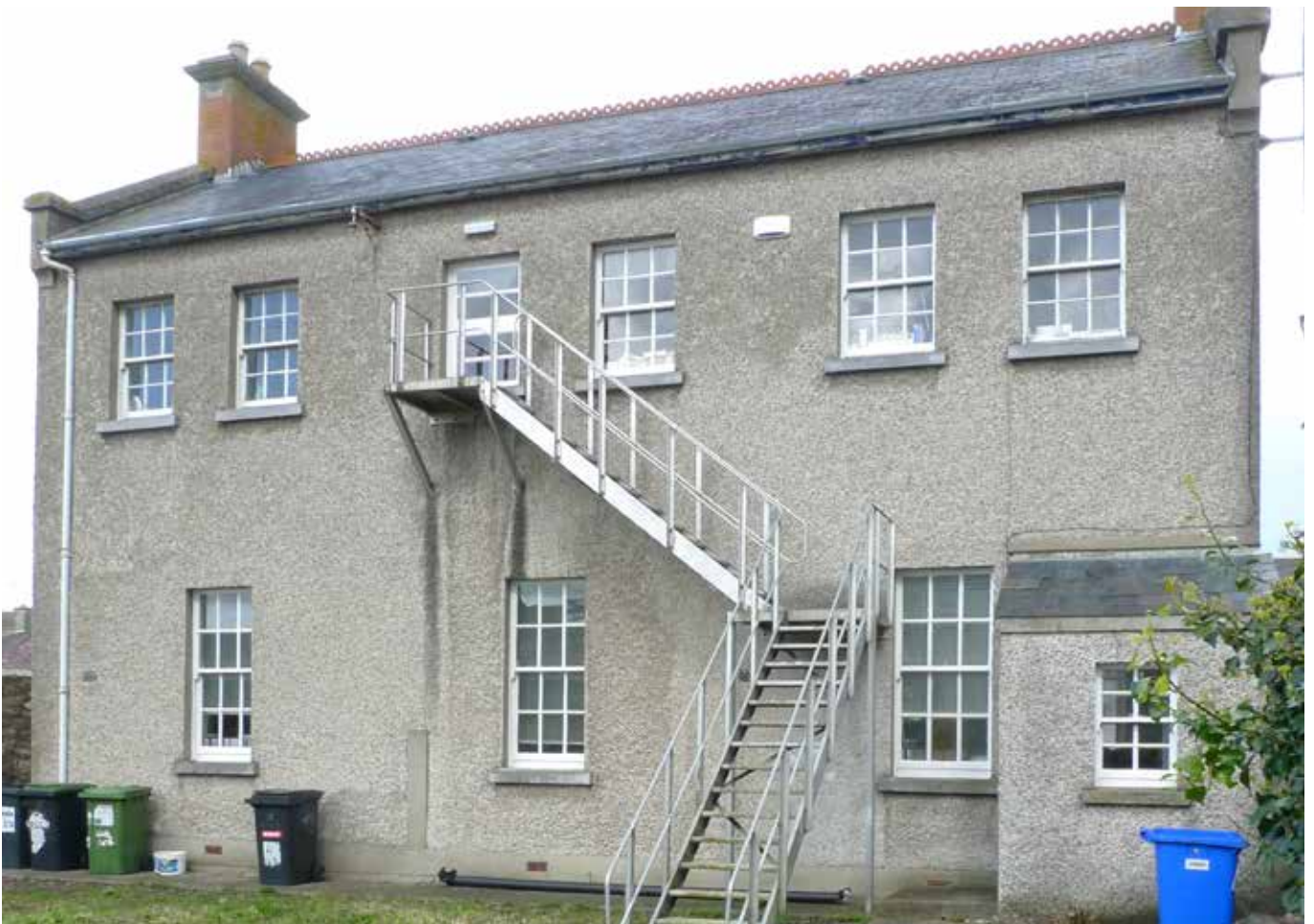
The rear facade of Skerries Library. The large iron fire escape stairs is very intrusive. It is also substandard in terms of access to it and being located over a window. It is suspected that, with a proper fire engineering approach a fire escape stair may not be necessary. If one is deemed necessary, it would be best located at a gable of the building.
