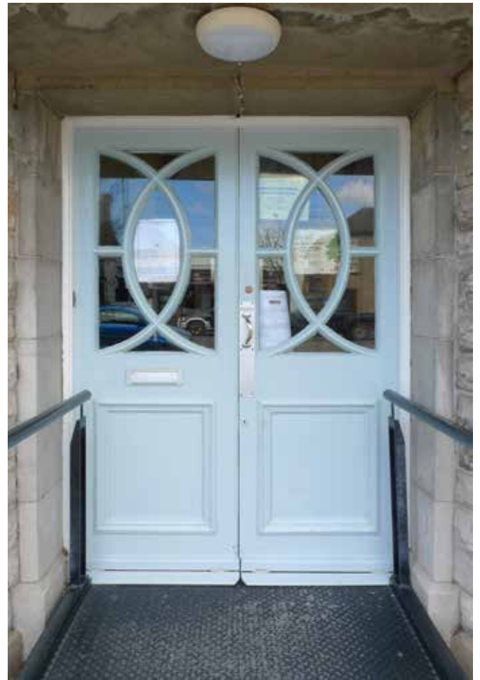
The fine original entrance doors. The door furniture might be reviewed.
