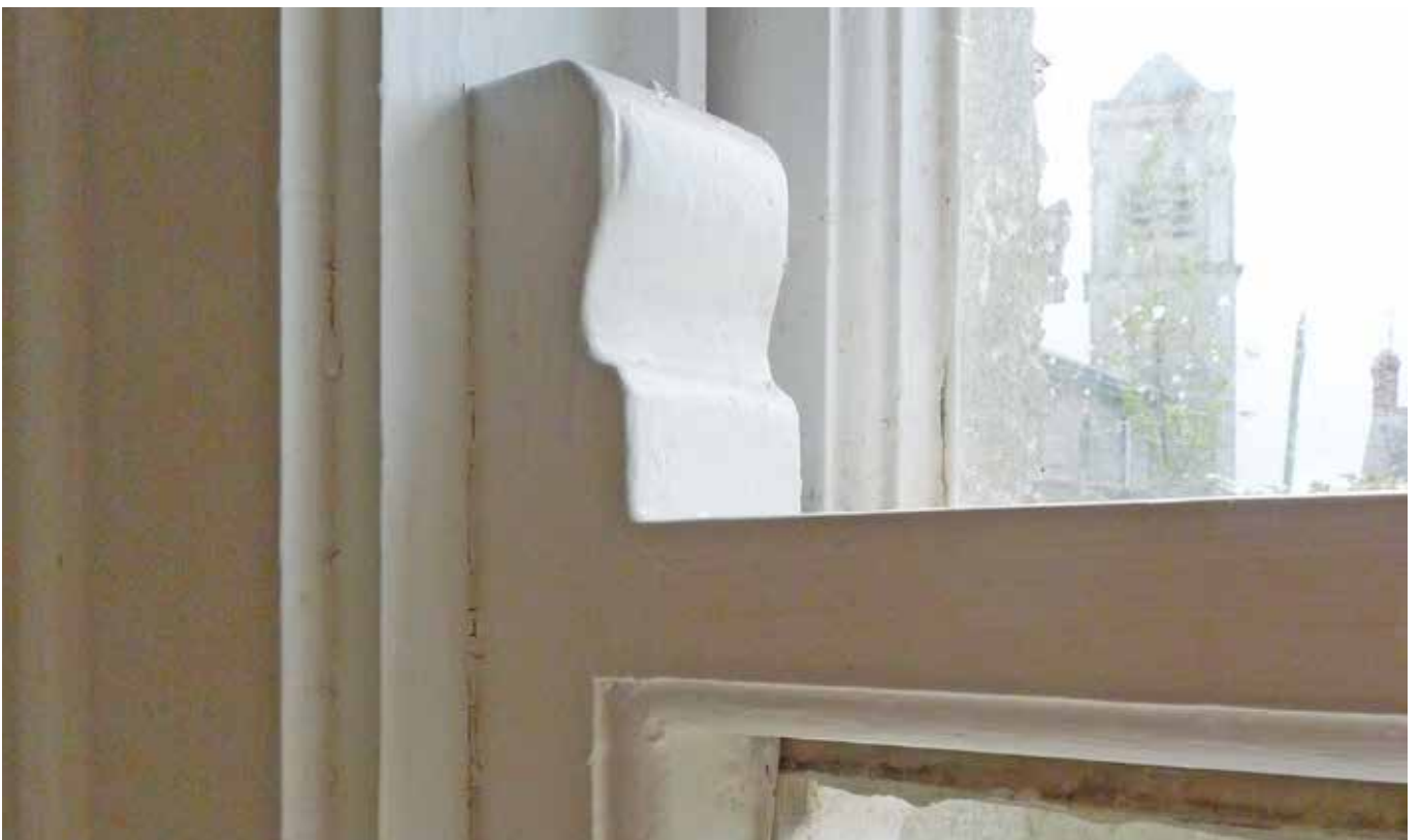
Detail of a typical sash window in Skerries Library
