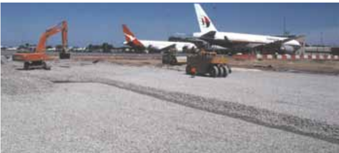
New taxiway at Adelaide Airport (Australia)
