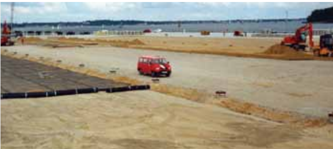
Tensar geogrids are perfect for dockside paving (Latvia)
