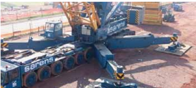
Heavyweight crane on Tensar ground stabilised working platform
