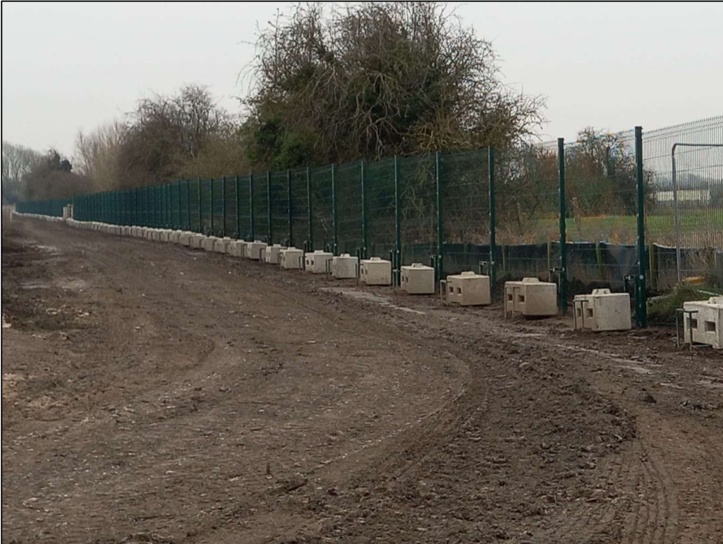
Figure 6 Example of temporary fence with supports
