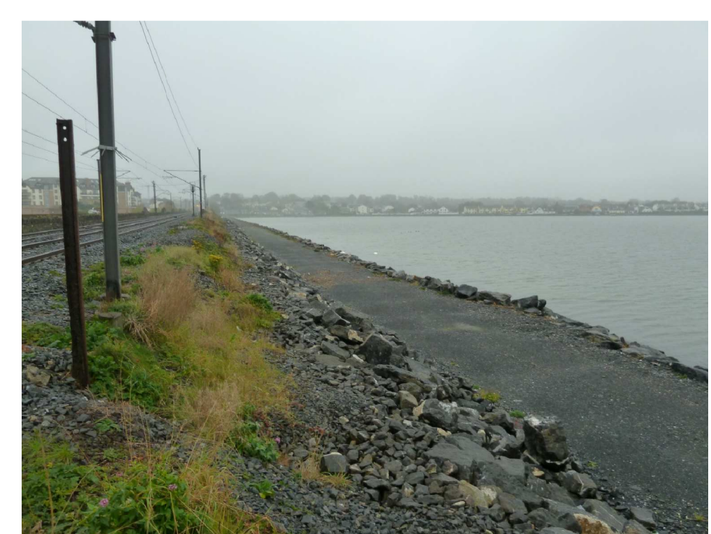
PHOTO 2 - EXISTING WEIR MAINTENANCE TRACK
