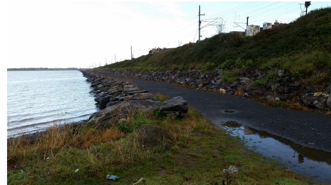
PHOTO 1 - EXISTING WEIR MAINTENANCE TRACK
