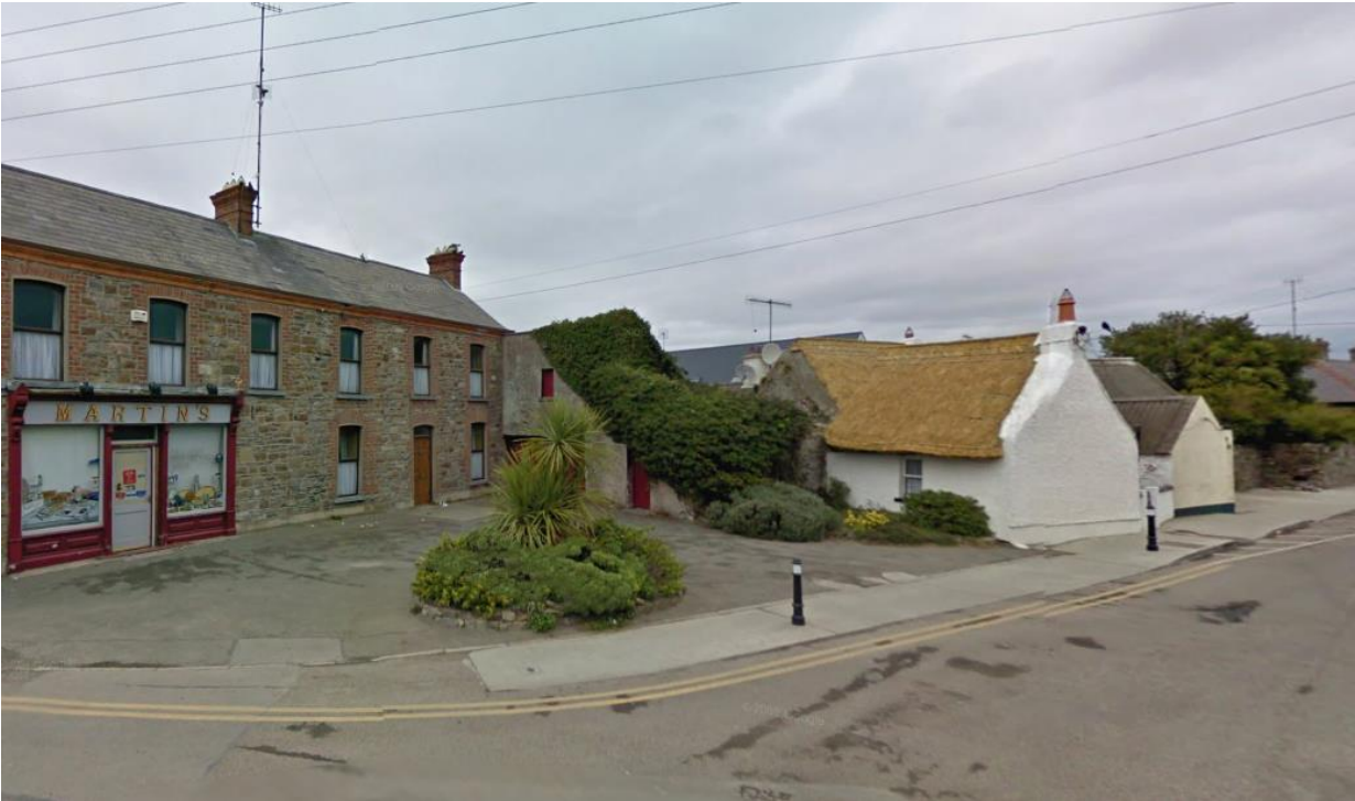
Fig 2: View of building showing derelict outbuilding structures (since demolished for Health & Safety reasons)
