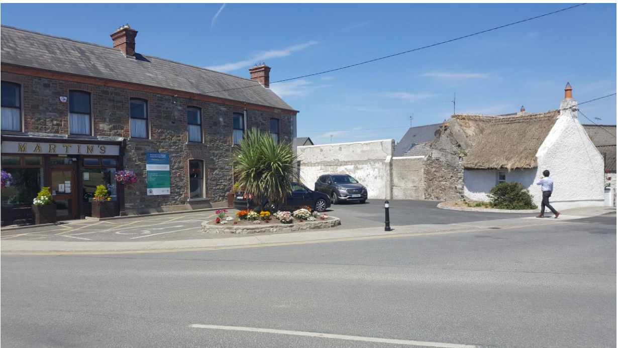
Fig 3: Current view of building with outbuilding structure demolished and exposed rendered boundary wall
